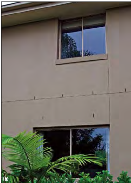
Figure 8 Articulation joint at window openings with masonry between
