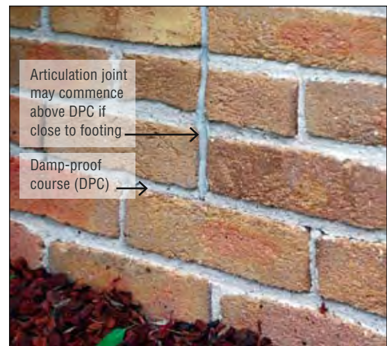
Figure 2 Articulation joint above damp-proof course
