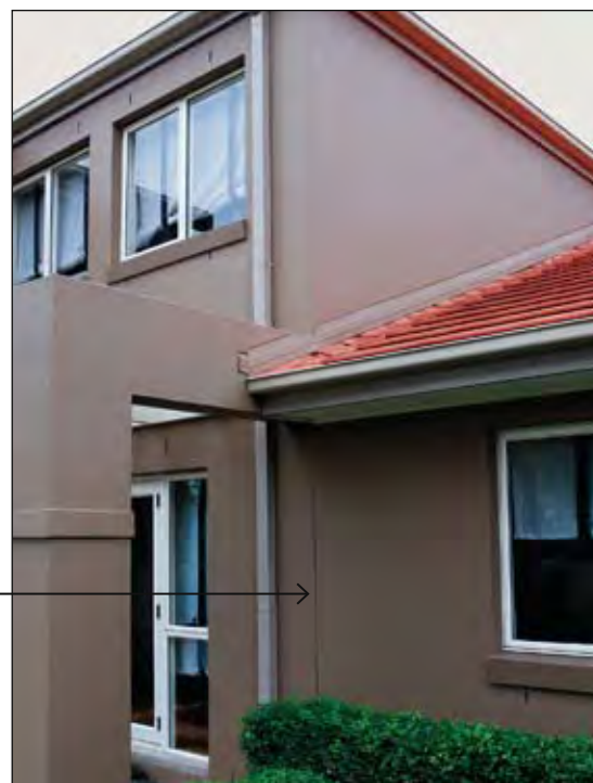
Figure 5 Articulation joints at changes of wall height
