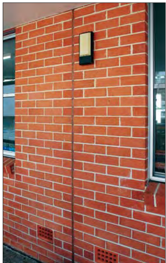
Figure 27 Articulation joint between openings
