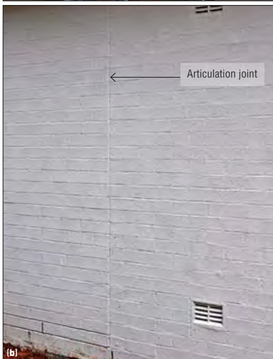
Figure 18 Joints should be continuous through applied finishes
