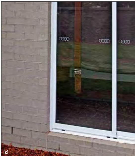
Figure 6 Articulation joints at window/door openings
