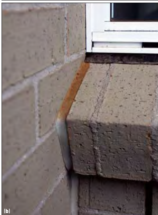
Figure 26 Articulation joints should be continuous (a) Joint should be continuous alongside window sill (b) Joint is continuous alongside window sill but required gap between masonry and window frame has not been provided
