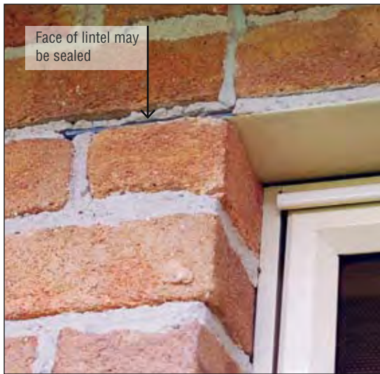
Figure 22 Bed joint along lintel may also require sealing at articulation joints
