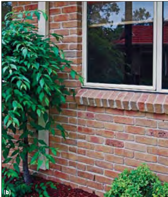
Figure 7 Articulation joints at window openings with infill panel between
