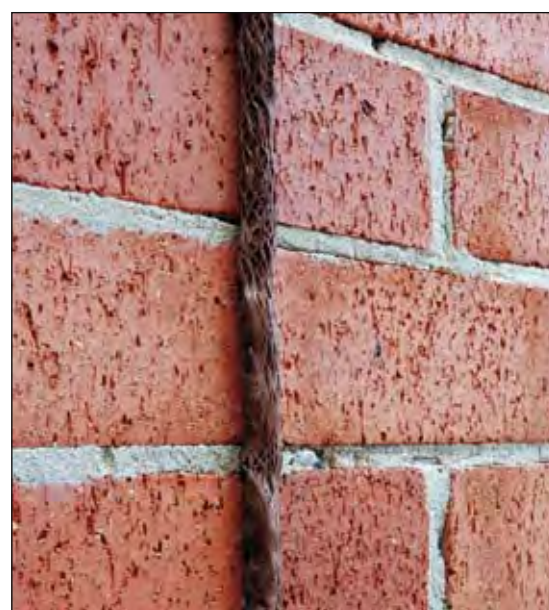
Figure 21 Joint filler/sealant squeezed out of joint as a result of not having been recessed
