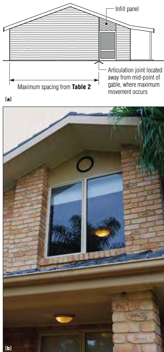
Figure 30 Articulated masonry gable-end wall (a) Location of articulation joint (b) Use of infill panels above openings
