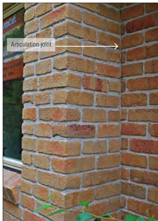
Figure 16 Articulation joint at offset in wall
