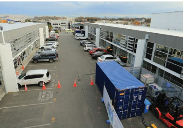
Commercial offices re-levelled while occupied
