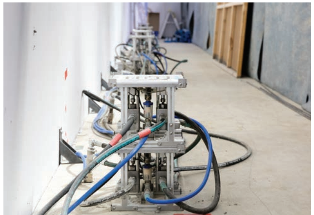
Re-levelled 165mm
