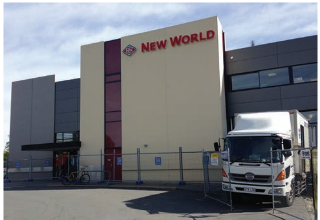
Supermarket re-levelled 180mm
