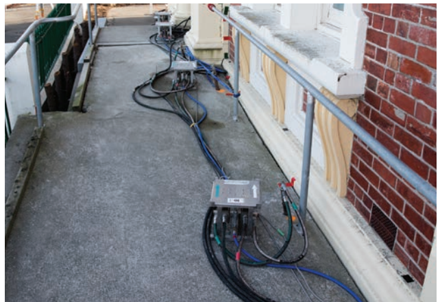
1833 building re-levelled 240mm
