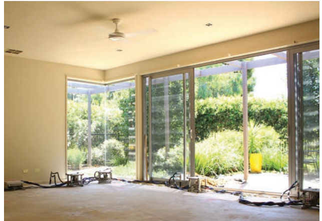
Entire home re-levelled 175mm
