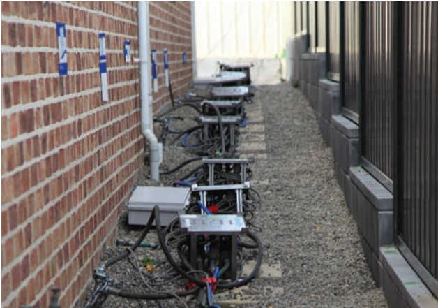
Home re-levelled while occupied
