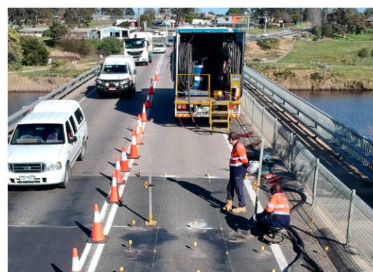
Minimal road disruption during injection works
