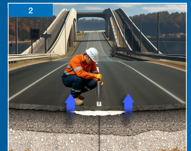
Teretek® resin is injected into the treatment zone filling voids and compacting weak soils.
