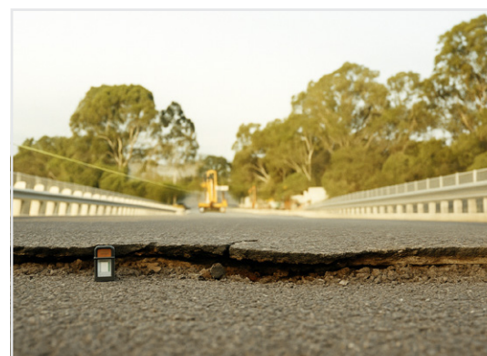
Raised approach slab ready for profiling
